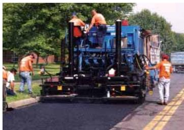
Micro-surfacing applies a durable, polymer-modified asphalt seal to roads that have begun to show signs of aging and minor distress. By retarding the surface's natural breakdown, this process extends the highway's lifespan six to eight years.
