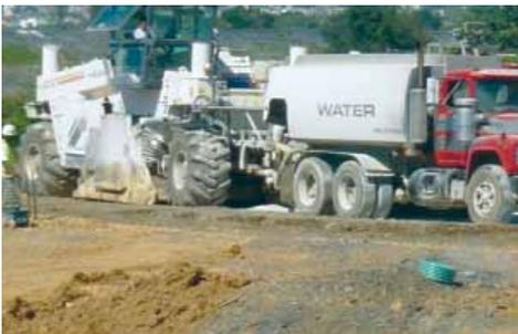
Because Full Depth Reclamation reuses 100% of existing road material, no material is exported from the project site and land-filled or discarded as backfill. Roadways that have cracked and deteriorated as a result of poor sub-base structure can be completely reconstructed and strengthened. It is the perfect solution for rebuilding weakened pavements for highways, parking lots, airfields and industrial sites.
